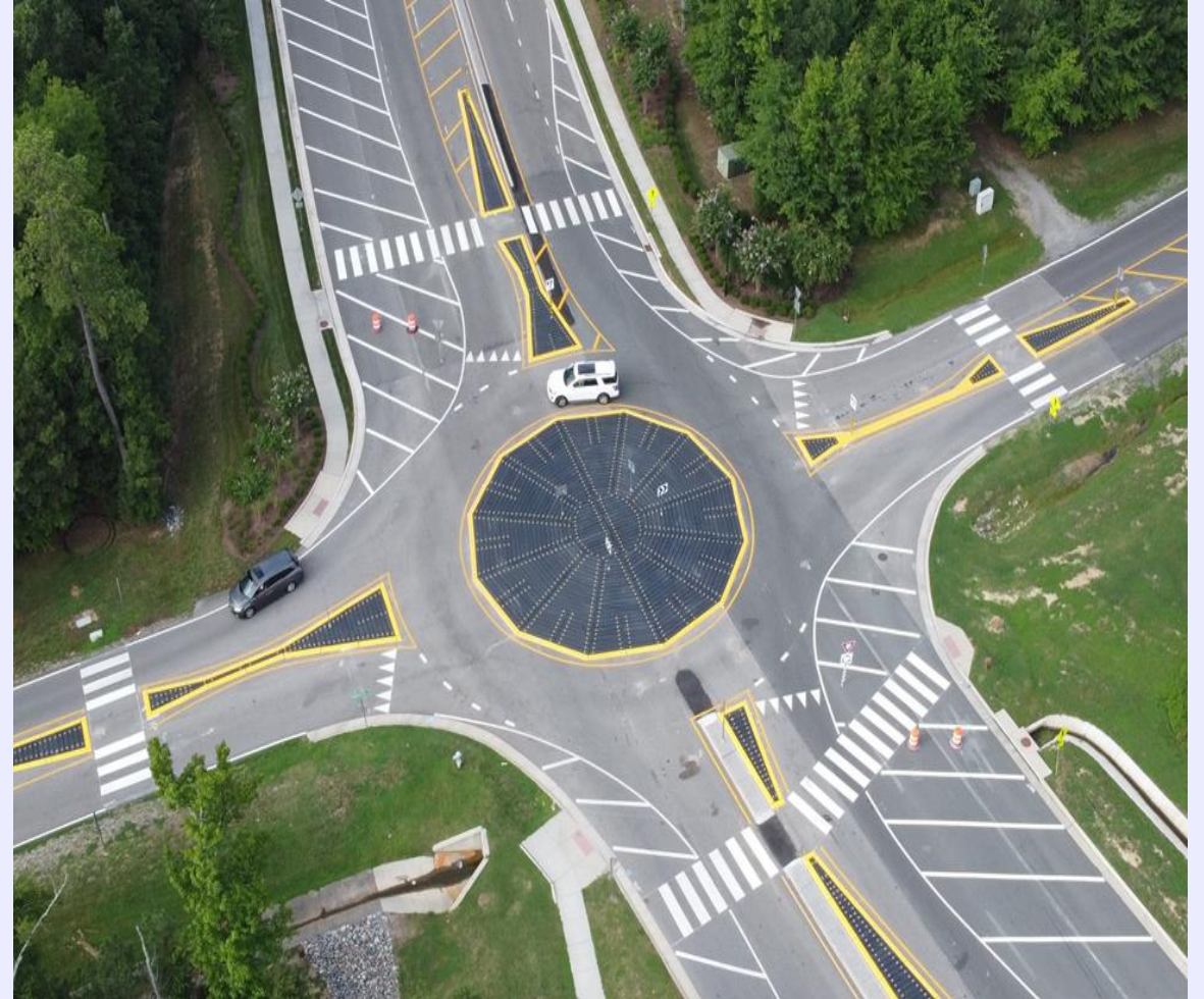
Photo of Vortex roundabout, Annandale, Va. courtesy of ZKxKZ Vortexroundabouts.com
